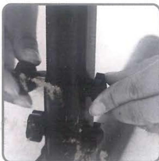
The base support rod is installed
